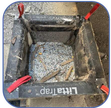
Plastic pellets captured a storm drain screens with a 1 mm liner deployed on the properties of plastic companies.
