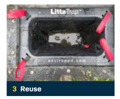
Reuse the Litta $Trap^{\mathsf{TM}}$  by placing securely back into the surrounding frame and seal, and close grate.
