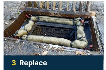
Once the LavaSorb™ boom basalt fibres are saturated, they can be wrung out with a wringer and the booms can be placed back in the pit with approximately 90% of the original capture volume. Otherwise, the booms can be disposed of according to local regulations.
