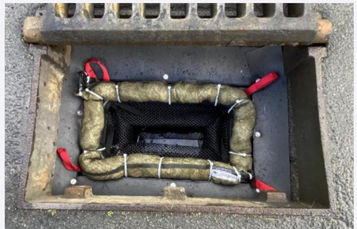
LavaSorb™ Boom set up with EnviroPod™ LittaTrap™ to ensure it absorbs the oils and oil-based liquids.
