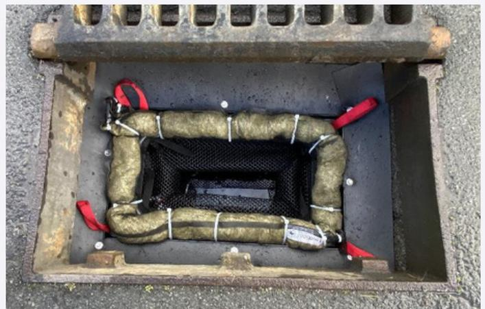
LavaSorb™ boom set up with EnviroPod200™ to ensure it absorbs oils and oil-based liquids in the stormwater.
