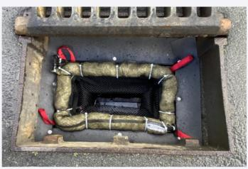
LavaSorb<sup>™</sup> boom set up with EnviroPod200<sup>™</sup> to ensure it absorbs oils and oil-based liquids in the stormwater.
