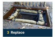
Once the LavaSorb<sup>™</sup> boom basalt fibres are saturated, they can be wrung out with a wringer and the booms can be placed back in the pit with approximately 90% of the original capture volume. Otherwise, the booms can be disposed of according to local regulations.
