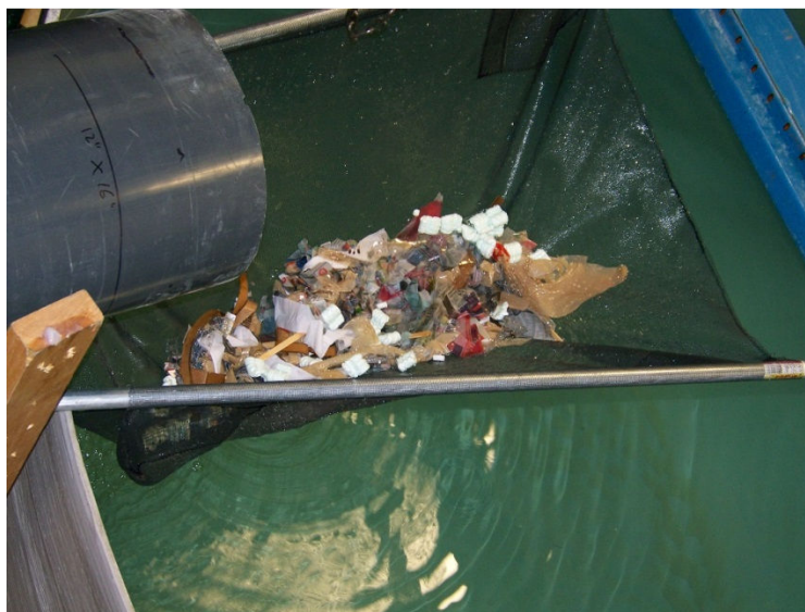
Figure 12: Escaped Solids – Control at 15 L/s
