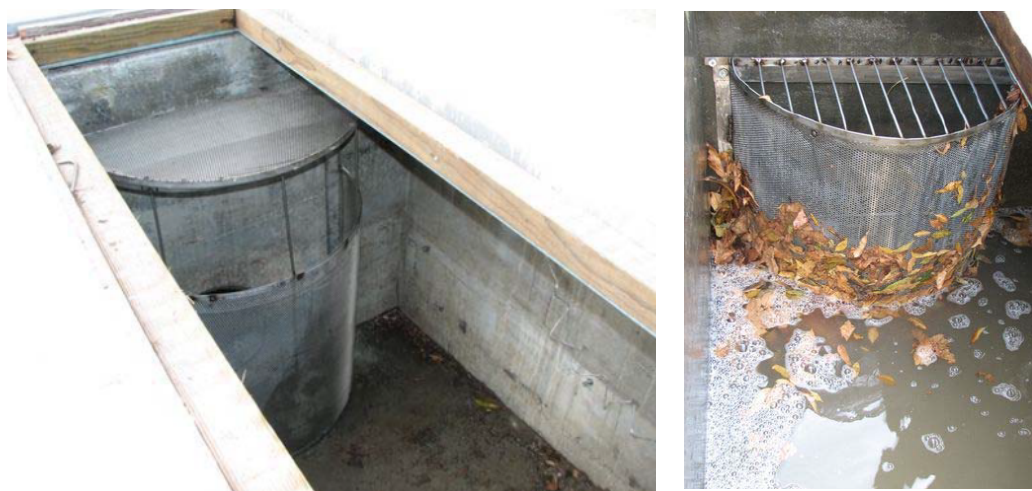
Figure 7 Images from the County of Los Angeles Department of Public Works Technical Report entitled Connector Pipe Screen Full Capture TMDL Compliance Screen and bypass sizing requirements (Moon, 2007).
