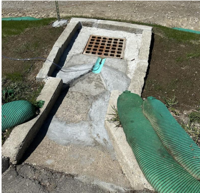
Figure 6. Influent sluice and catch basin at UNH. The sample line set in the concrete sluice forms the influent sampling point; granite curbing directs runoff into the basin.
